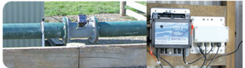
Irrigation Watermeter Installation
