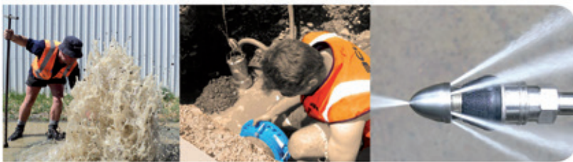
Pipe & Drain Repairs & Unblocking
